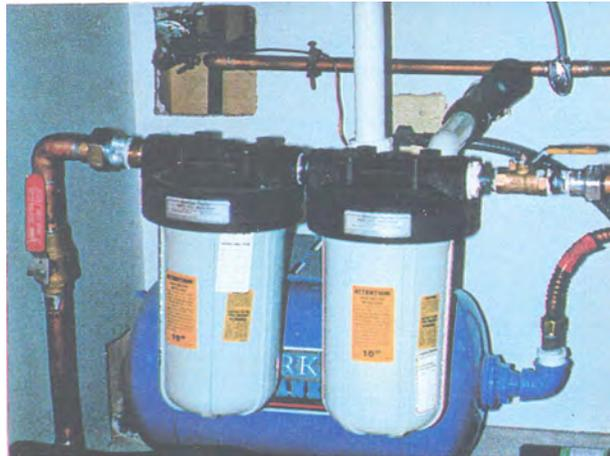
Fig. 7.6 10 micron and 0.5 micron filters
